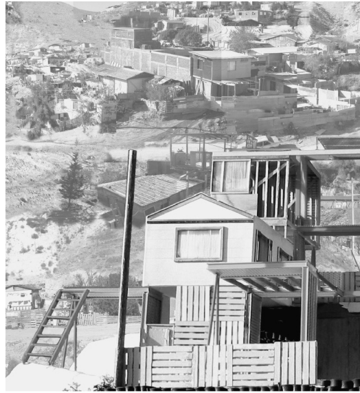
FIGURE 6. A housing innovation made of waste: A maquiladora-made prefabricated frame performs as a hinge mechanism to connect a variety of recycled materials and systems brought from San Diego and reassembled in Tijuana's slums.
